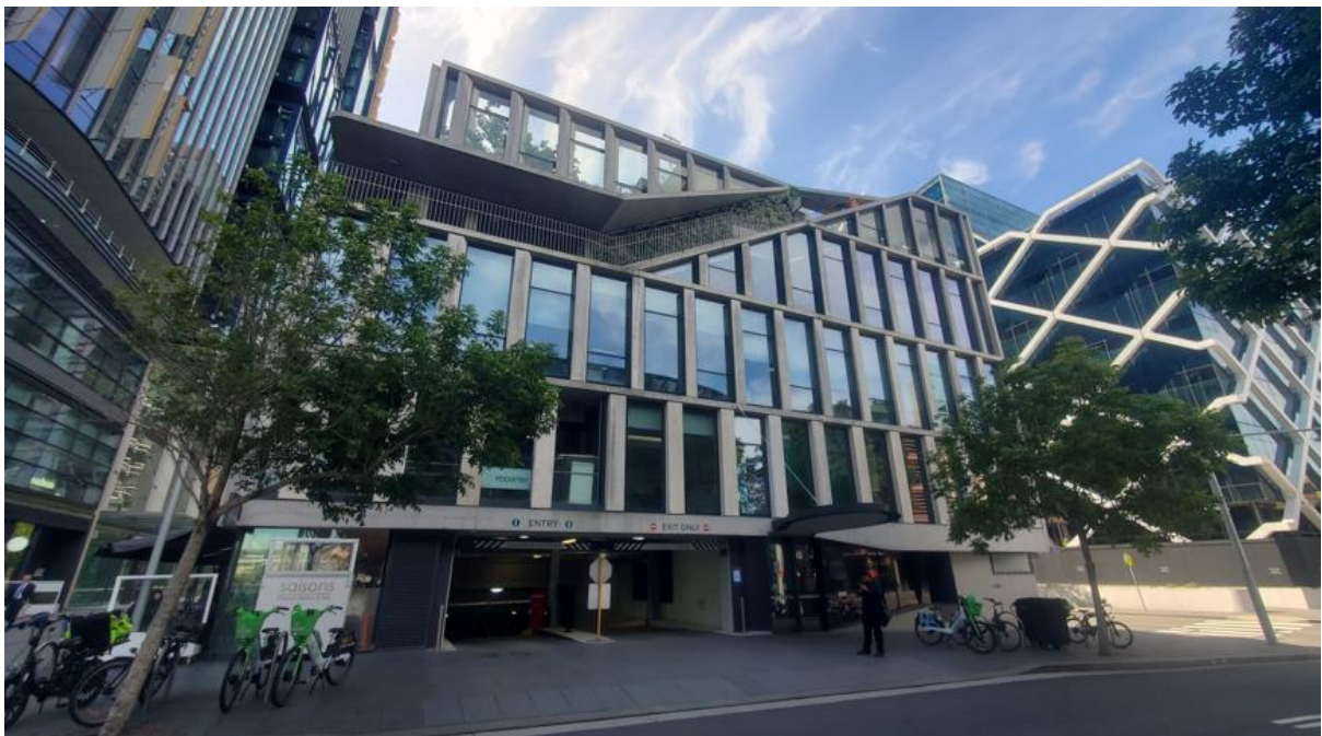
Figure 4: Site viewed from Barangaroo Avenue facing east
