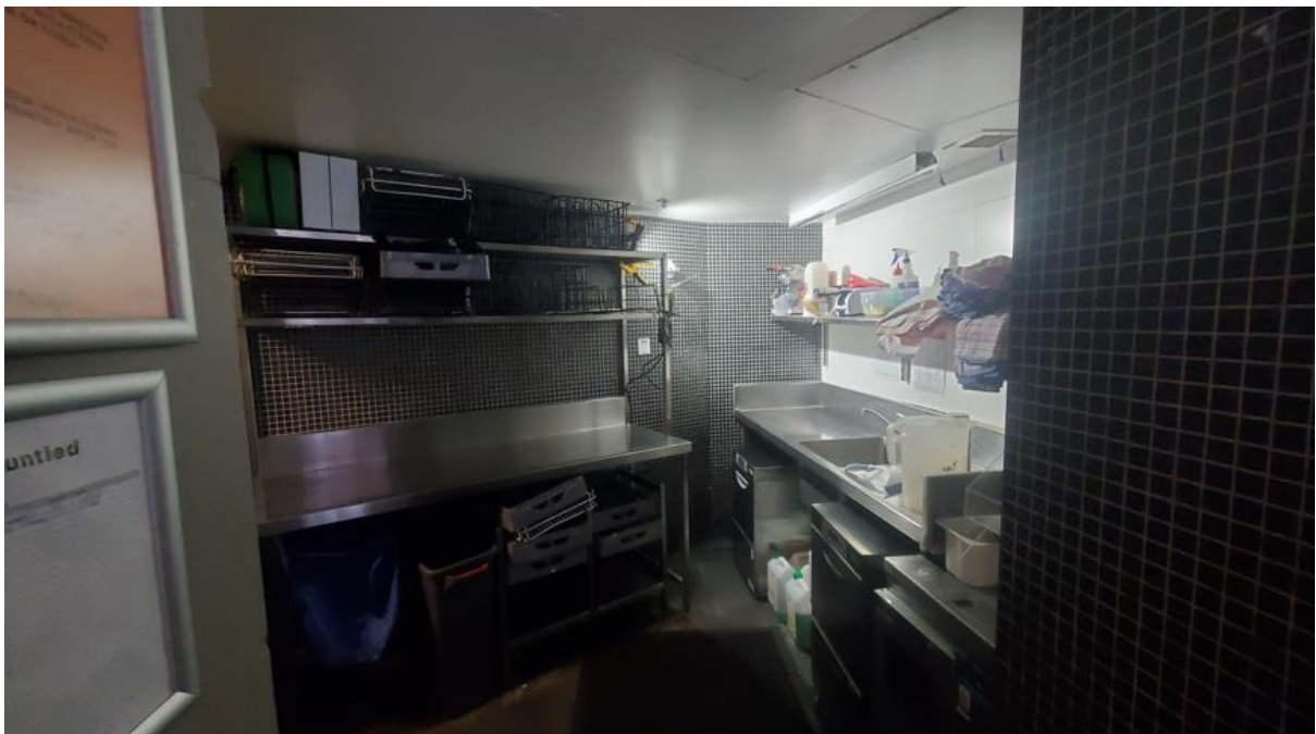
Figure 16: Part of existing kitchen
