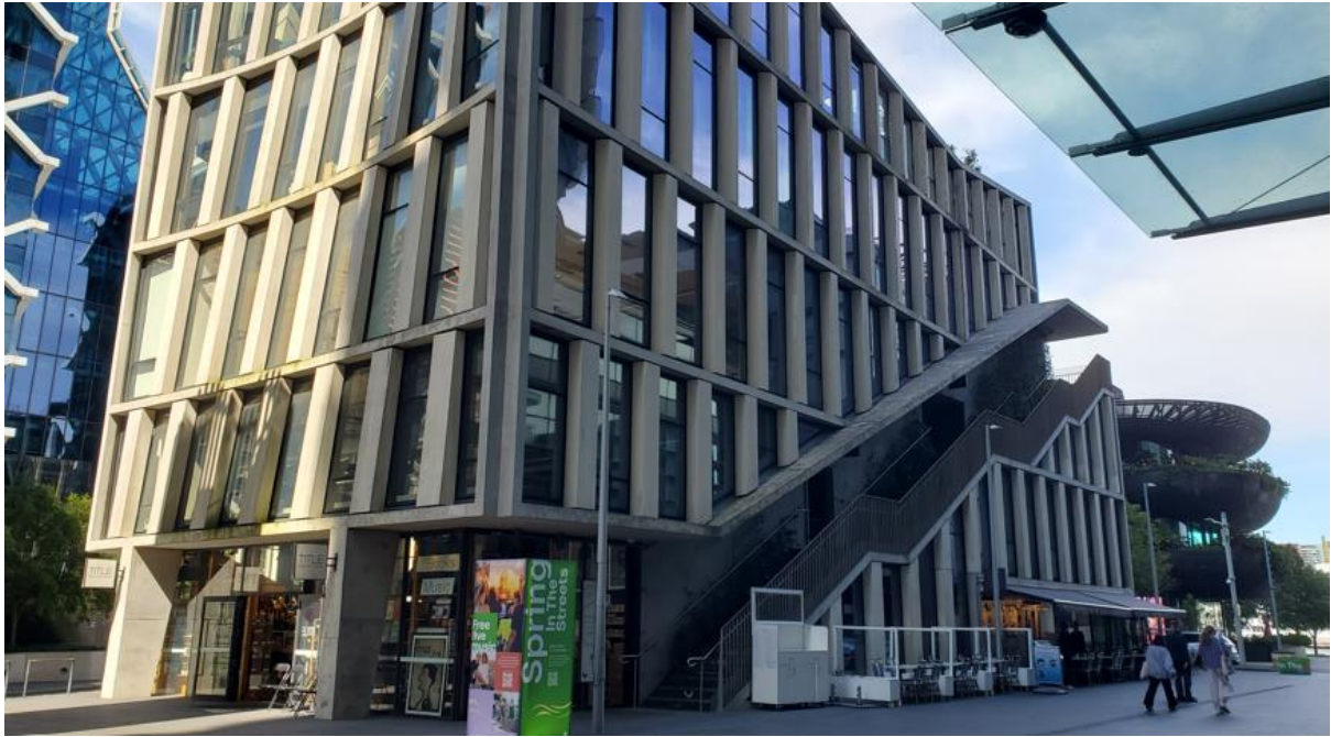
Figure 3: Site viewed from Exchange Place facing southwest
